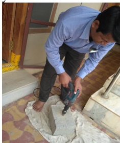
Fig.7 (a): Drilling the Blast Hole in F.A.B
