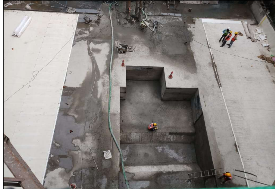
Fig 2: Freshly Poured Concrete near Blasting Sites at Mumbai Metro Rail Project
